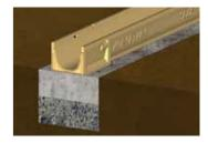
5. Position channel string, sump unit and end cap on the concrete bed.
